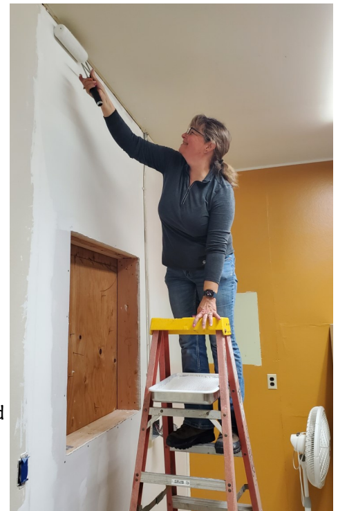
Tricia Cottrell touches up the wall above the kitchen window box.
